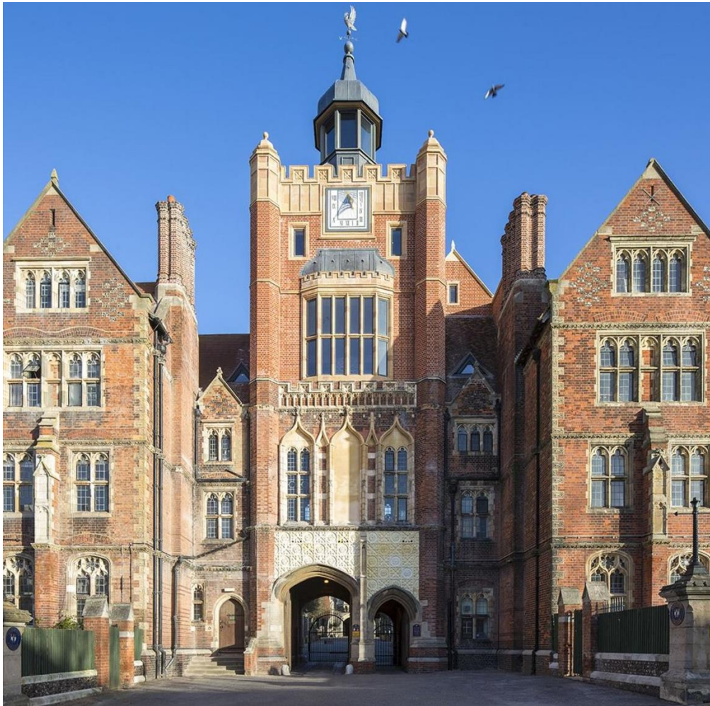
The gateway and clocktower before and after the work to complete the original design of the building was completed in 2014.
